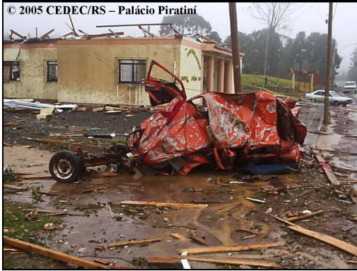
Figure 6: Destruction likely caused by a tornado in Muitos Capões, in Rio Grande do Sul State (southern Brazil) on 29 August 2005. Picture taken by a state CD official during the damage survey. (Courtesy of CD System of Rio Grande do Sul State.)
