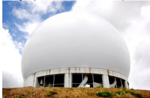
Figure 4. CP2 site infrastructure at Redbank Plains. Antenna and pedestal are within an inflated radome mounted over housing for office, storage and transceiver.
