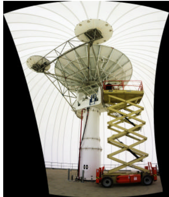
Figure 2. CP2 pedestal and antenna pictured during installation at Redbank Plains. Two X-Band cassegrain paraboloids are located above the primary centre fed S-Band paraboloid dish.
