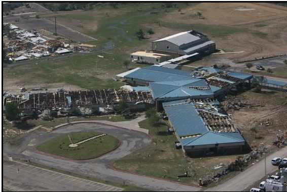
Figure 18. Aerial view of the Rosita Valley Elementary School looking southeast. This steel-framed structure lost a considerable amount of its metal roof and wall cladding.
