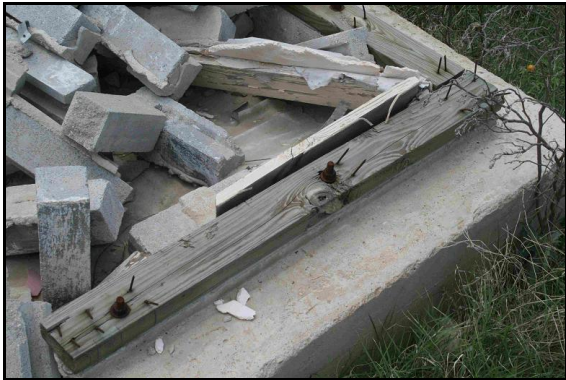
Figure 15. Failure of the wall framing occurred when the studs pulled out of their straight-nailed connections to the wall bottom plates. Note wall bottom plates were anchored to the concrete slab foundation.
