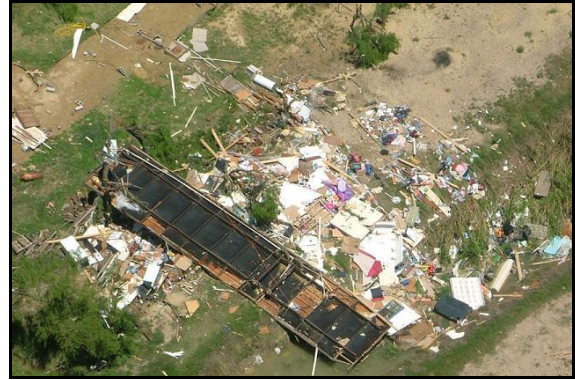
Figure 16. One of several flipped manufactured homes rated EF-2 (DOD=8). The original location of the home was in the upper left corner of the picture.
