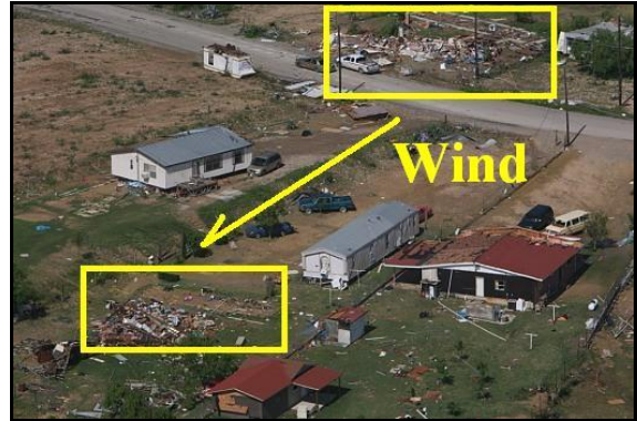
Figure 17. Variation in the performance of manufactured homes related to the orientation to the wind. Two manufactured homes (yellow boxes) were destroyed when broadsided by the strongest winds while other manufactured homes parallel to the wind remained.
