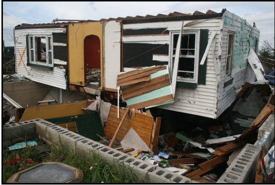
Figure 13. Unanchored home that slid off its CMU foundation was rated EF-2 due to loss of its roof.
