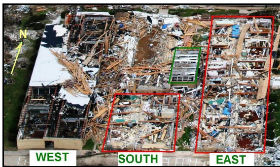
Figure 12. Aerial view of the Delmer Day Elementary School looking north. Unreinforced masonry walls (red outlines) collapsed to the west.
