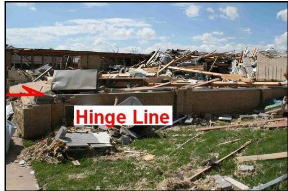
Figure 13. East wall of the South building toppled inward rotating about the base of the windows. Red arrow indicates hinge line.
