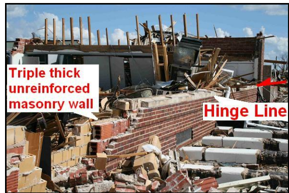
Figure 10. West wall of south wing fell outward rotating about the base of the windows. Red arrow indicates hinge line.
