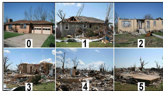
Figure 3. Examples of EF-scale damage ratings to homes in Greensburg, KS.
