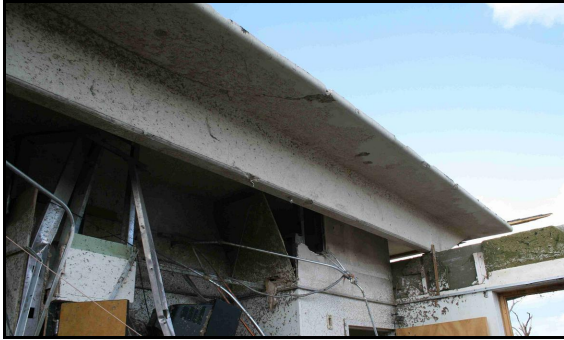
Figure 15. Wind removed a 4500 kg steel-reinforced concrete roof beam on the hospital.
