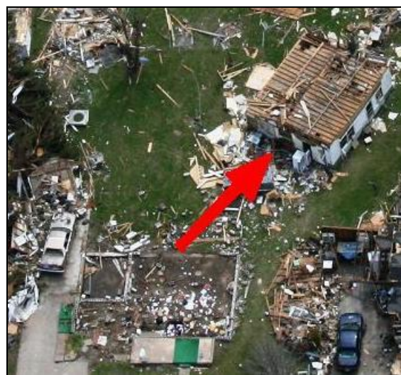
Figure 4. Example showing a home that was "swept clean" from its foundation that was rated EF-2 based on the removal of its roof. Note vehicle remained within the destroyed garage.
