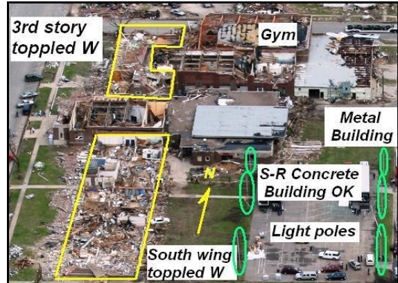
Figure 9. Aerial view of the Greensburg High School looking north. Unreinforced masonry walls collapsed (yellow outlines) to the west whereas the steel reinforced concrete building remained intact.
