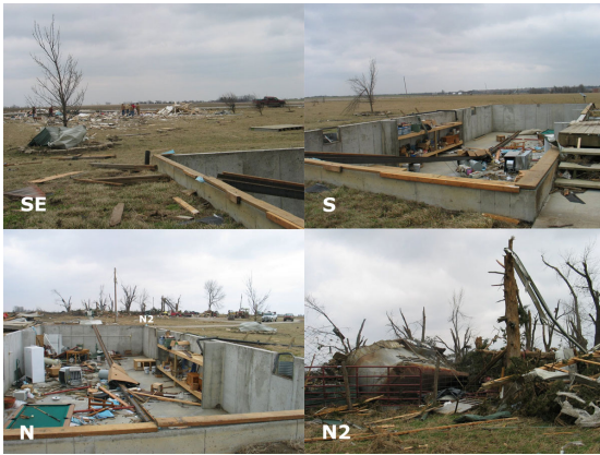
Figure 8. A house (FR12) experienced DOD=10 next to two saplings (TH) experiencing DOD<3. More mature trees experienced DOD=3 to 5 north of the house (bottom two panels). This image is provided courtesy of Evan Bookbinder NWS EAX.
