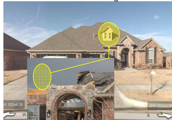
Figure 5. A surveyed house exhibited total failure of its roof on 31 March, 2008. A Dormer window is highlighted by the orange oval in the picture of the house before the damage occurred. The background picture is courtesy of Google while the damage picture was taken by Kiel Ortega.
