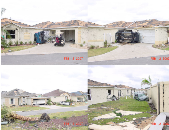
Figure 3. Four houses (DI=FR12) with displaced vehicles taken from Lady Lakes, FL (Photographs courtesy of NWS Tampa).
