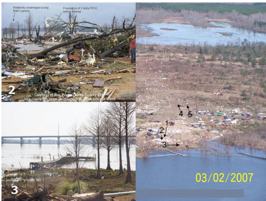
Figure 8. Damage at Millers Ferry, AL from 01 March, 2007. At right is an aerial picture facing northeast. The numbers correspond to photos including #2 (upper left) and #3 (lower right). The aerial photograph is taken courtesy of NWS Mobile. Photograph #2 is taken by Roy Waite. Photograph #3 is taken by Jim LaDue.
