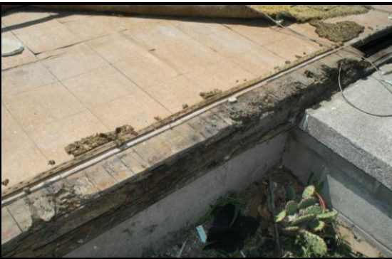
Figure 11. Rot and termite damage to perimeter flooring beneath where the wall bottom plate had been located.
