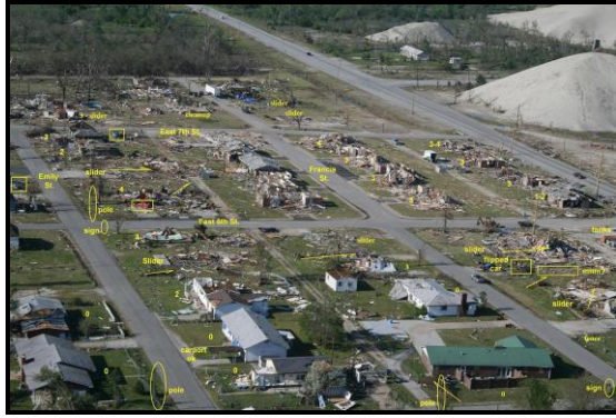
Figure 5. Aerial view of the tornado damage path looking south, just east of Highway 69. Pertinent features are noted. Chat piles are to the right.
