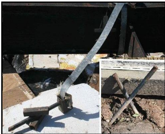
Figure 14. Failure of rock type anchor on a manufactured home. The anchor remained strapped to steel I-beam. The inset image show crossed steel rods remained in the ground.
