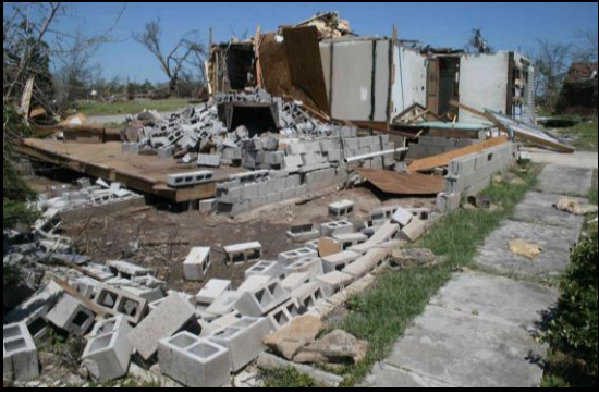
Figure 9. An unanchored home that slid off its pier and beam foundation.
