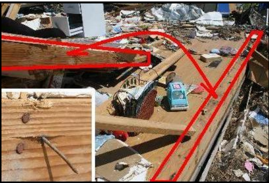
Figure 10. Bottom plate of the wall (left) failed where it was nailed to the floor perimeter (right). The inset image shows a nail that extended from the bottom plate.
