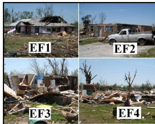
Figure 7. EF-scale numbers assigned to homes in Picher based on the increasing severity of the damage.
