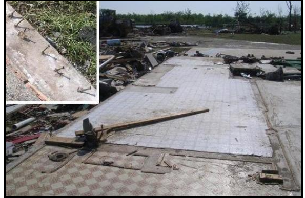
Figure 12. A poorly anchored home swept clean off its concrete slab foundation. The inset image shows nails along foundation perimeter (NOAA).
