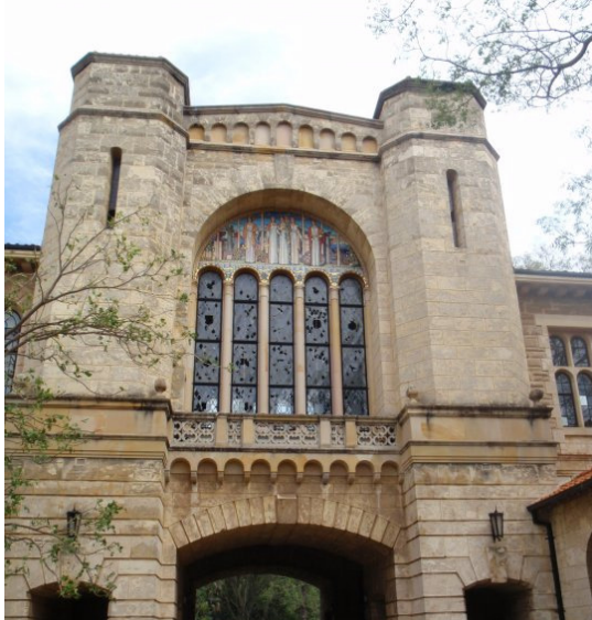
Figure 11: Photograph of 6cm hail damage to 80 year old stained glass windows at Winthrop Hall at the University of Western Australia.
