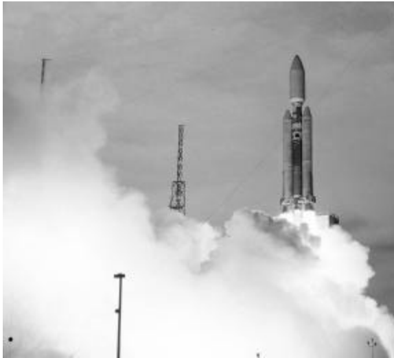
Figure 2 Lightning protection masts and overhead protective grid for the Titan IV launch pad at CCAFS.
