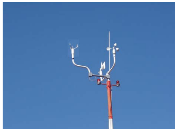
Figure 4. ASOS wind tower with dual installation of Belfort 2000 and 425NWS
