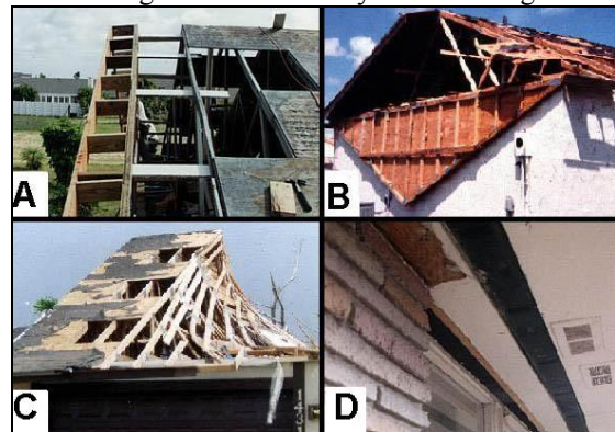
Figure 2. Examples of wind damage to the roof structure: A) removal of decking, B) failure of gable end, C) rotation of trusses, and D) shifting of a roof due to tree impact.
