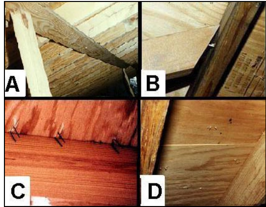
Figure 1. Inherent deficiencies in roof construction not related to wind: A) sagging of rafters due to inadequate support, B) gap between rafter and ridge beam from poor joinery, C) deck staples that missed the rafter, and D) wavy roof deck from lack of clips.
