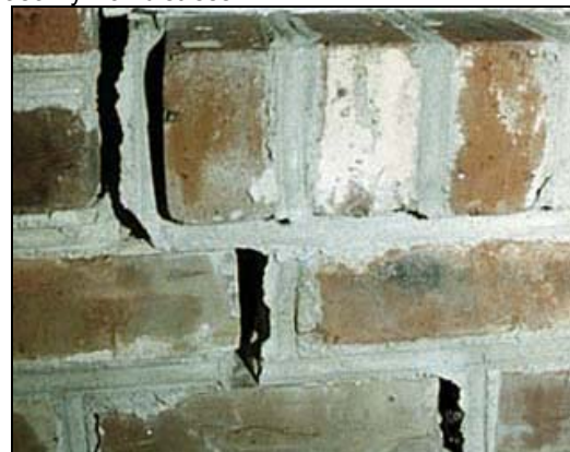
Figure 15. Stair-step crack in brick masonry from differential foundation movement. This distress was not caused by the tornado.
