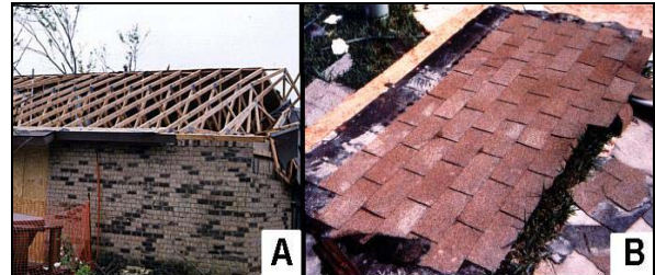
Figure 7. Examples of wind damage to roof decking: A) Loss of entire roof deck since it was not fastened to the trusses, B) entire deck sheet with shingles still attached.
