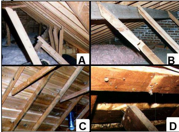
Figure 9. Wind damage to the roof structure: A) failed nailed connections where purlins were attached to rafters, B) broken brace, C) failed nailed connections between collar beams and rafters, and D) failure of nailed connection where brace was attached to purlin.
