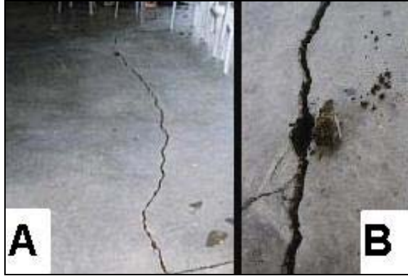
Figure 21. Cracks in concrete slab not caused by wind: A) center crack and B) close-up view showing dirt in crack.
