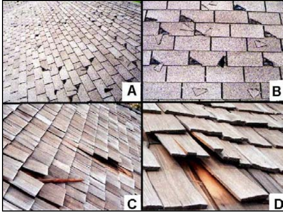
Figure 4. Intentional mechanical damage to roofs in attempt to simulate wind damage: A) torn tab corners upslope away from roof edge, B) closer view showing tab pieces remaining on roof, C) uplifted shakes, and D) closer view of uplifted shakes.
