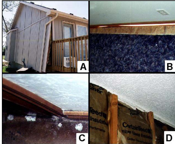
Figure 12. Examples of wall failures due to wind: A) base of wall pushed outward, B) failure of bottom plate to wooden floor connection, C) failure of bottom plate to concrete slab connection, and D) failure of wall stud to top plate connection.
