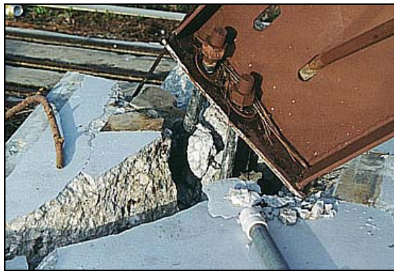
Figure 22. Cracks in concrete slab caused by the rotation of the steel column that failed in the wind.
