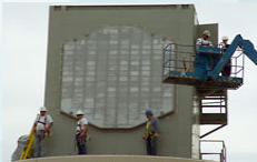
Fig.1 The NWRT antenna is being installed at Norman, Oklahoma
