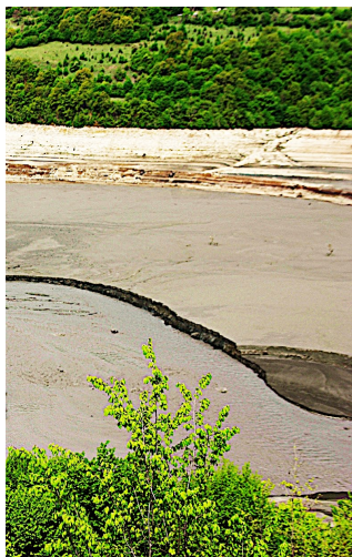
Field research: general view of mountain reservoir's silting prism
