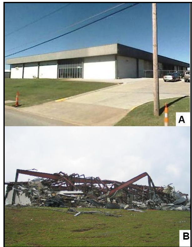
Figure 28. Southeast elevation of the Cummins Equipment building: a) before and b) after the tornado. This steel-framed structure had non load-bearing CMU curtain walls that collapsed during the tornado.
