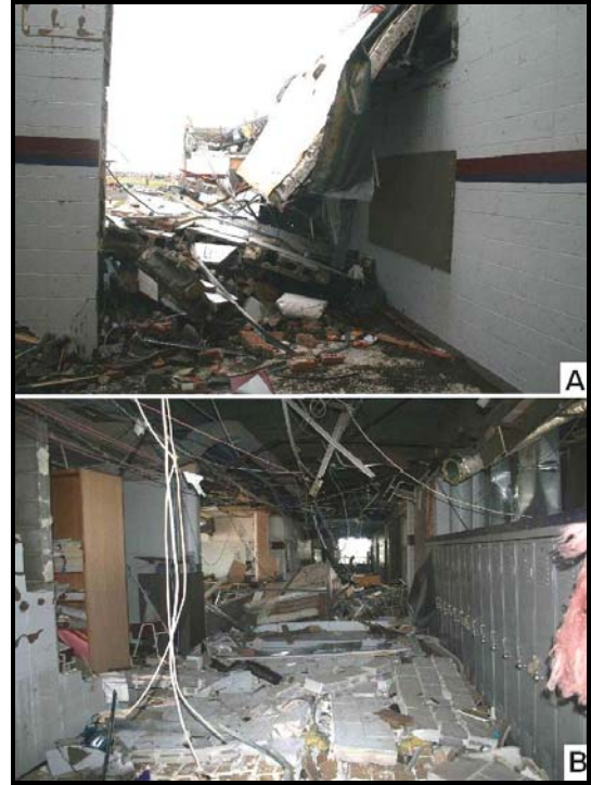
Figure 21. Collapse of second story CMU walls at the Joplin High School: (a) north hallway and (b) center hallway.
