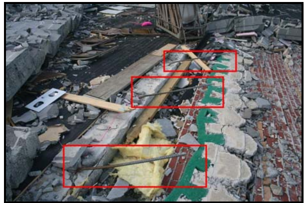
Figure 19. Base of the east auditorium wall showing foundation rebar (red boxes) bent to the east. This wall had little resistance to lateral wind pressures.
