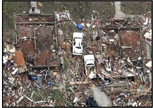
Figure 4. Homes swept clean from their pier and beam foundations. Note the vehicles remained.
