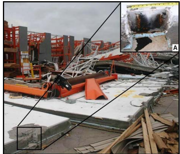
Figure 13. Toppled wall panels on the east side of the Home Depot building. Inset view (a) is a close up of a wall pocket where welds failed that attached the ends of the steel roof joists.
