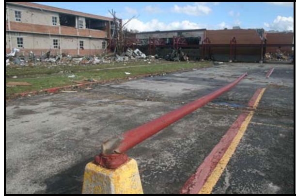
Figure 33. A light pole bent to the south in the High School parking lot.
