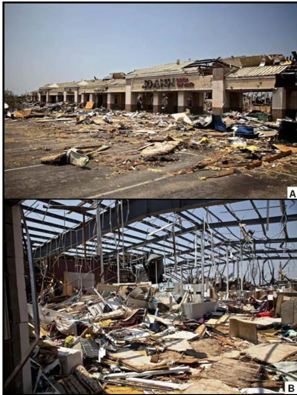
Figure 10. Front (east) elevation of the Bel-Aire Plaza Shopping Center. Tornadoic winds toppled the back (west) walls and removed the steel roof decking.
