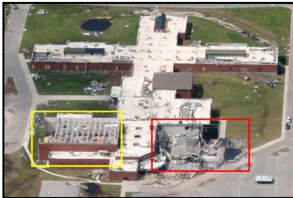
Figure 16. Aerial view of the East Joplin Middle School: (a) before and (b) after the tornado. The yellow box outlines the damaged gymnasium and the red box outlines the collapsed auditorium.
