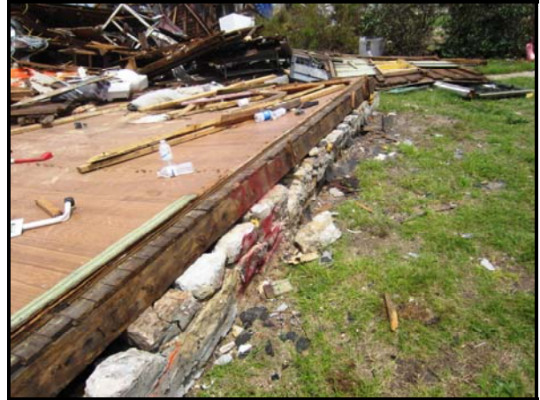
Figure 3. Floor platform supported by a rock masonry foundation.
