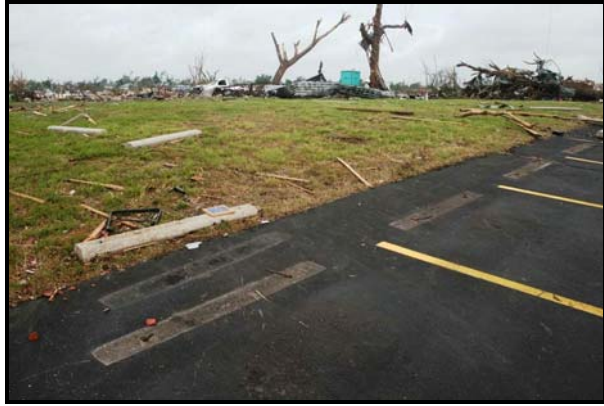
Figure 38. Removed concrete curbs (thrown westward) in a parking lot of a professional building just west of St. Johns Hospital.
