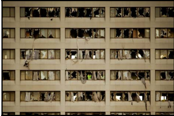
Figure 25. Loss of window glass on the north elevation of St. Johns Hospital.
