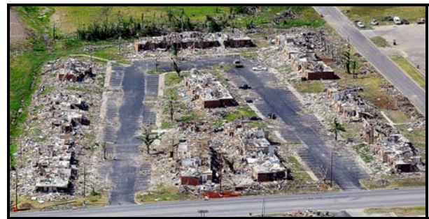
Figure 6. Aerial image of the Hampshire Terrace Apartments looking south. The tornado blew away the second story units. Workers already had cleared most of the debris from the streets.
