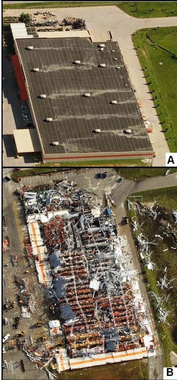
Figure 11. Aerial images of the Home Depot: a) before and b) after the tornado looking north. The superstructure collapsed when the wall panels toppled and the interior steel columns buckled.
