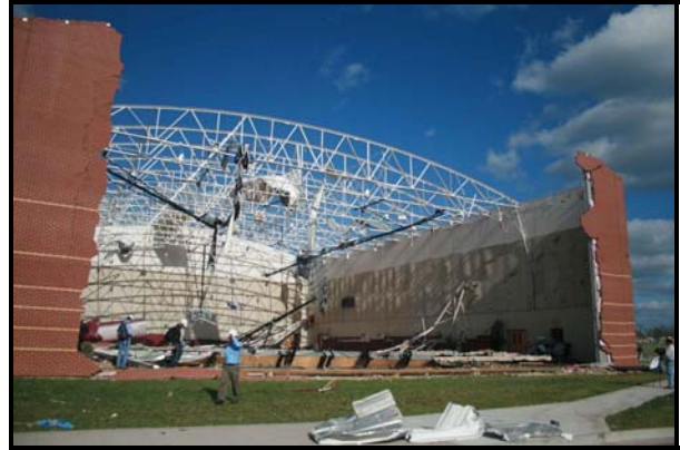
Figure 17. West wall in the gymnasium fell inward. The precast wall panels were attached poorly to each other and were not attached to the foundation.
