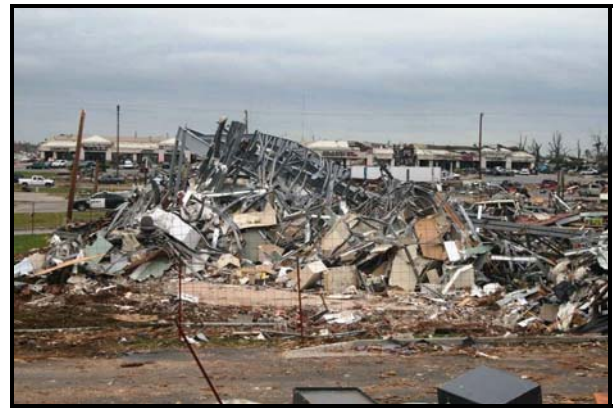
Figure 15. The center of the tornado passed directly over the Pennzoil Oil Change facility causing complete collapse of the building.
