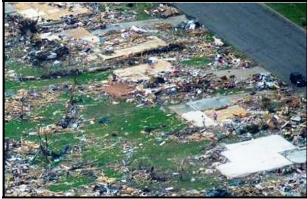
Figure 5. A row of homes swept clean from their concrete slab foundations were assigned EF-5 ratings.
