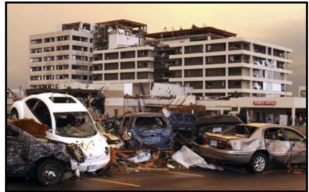
Figure 24. Northwest elevation view of St. Johns Hospital. The steel-framed structure remained intact. Cars were tossed around and crashed into each other in the parking lot.
