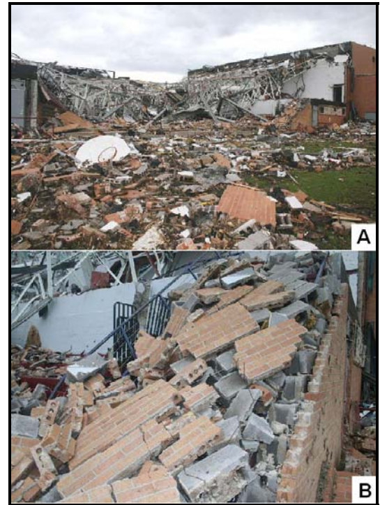
Figure 22. Collapse of CMU walls at the Joplin High School Gymnasium: (a) overall view looking east, and (b) close-up of the non load-bearing west which fell inward.
