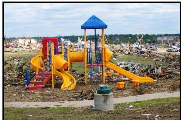
Figure 42. Child's play set was left virtually untouched in the middle of an EF-4/EF-5 area at Cunningham Park. Note the snapped steel pole in the foreground.
