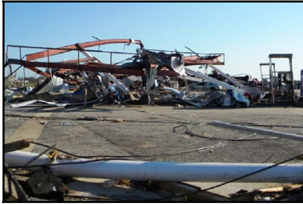
Figure 29. Collapse of a service station canopy in the Joplin tornado.
