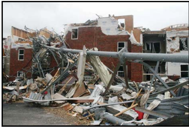
Figure 32. Cell phone tower toppled into one of the apartment buildings at the Plaza Apartments.
