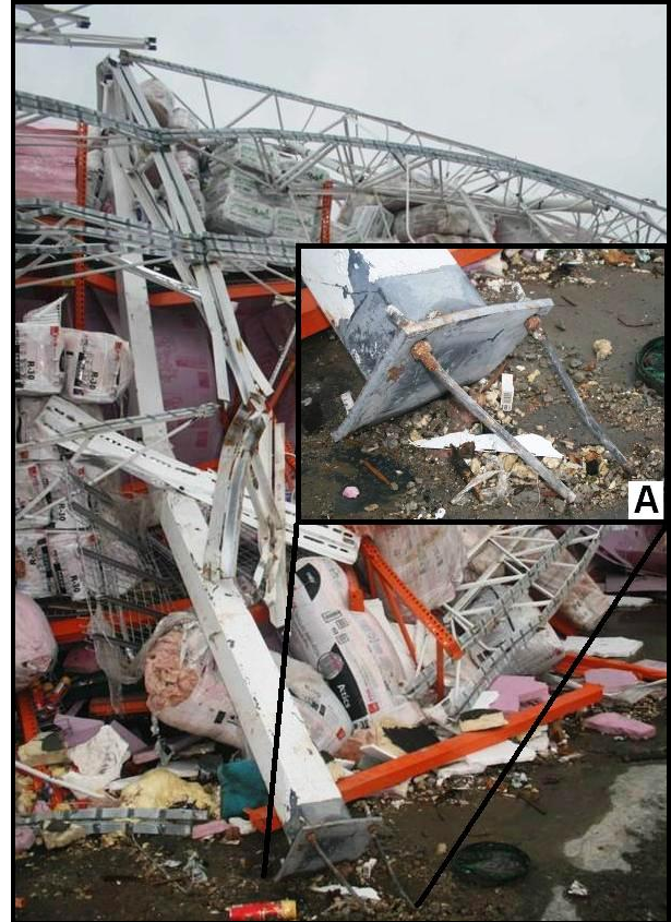
Figure 12. Base of a tubular steel column that failed when the anchor bolts pulled out of the concrete slab. Inset view (a) is a closer image.
