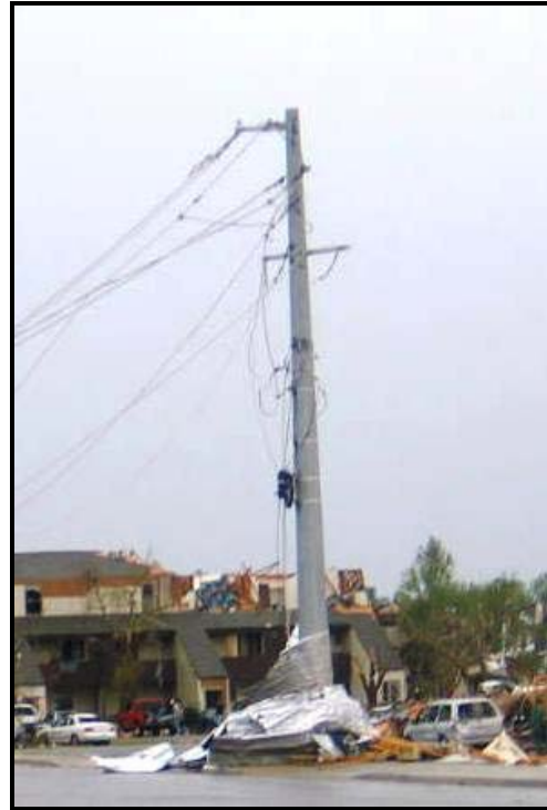
Figure 31. Damage to a tall, tapered steel pole that had supported power lines from the substation.
