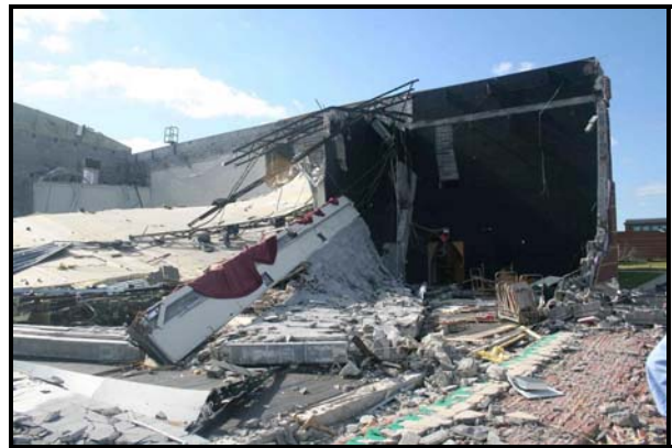
Figure 18. Roof on the auditorium collapsed when the south and east masonry walls failed.
