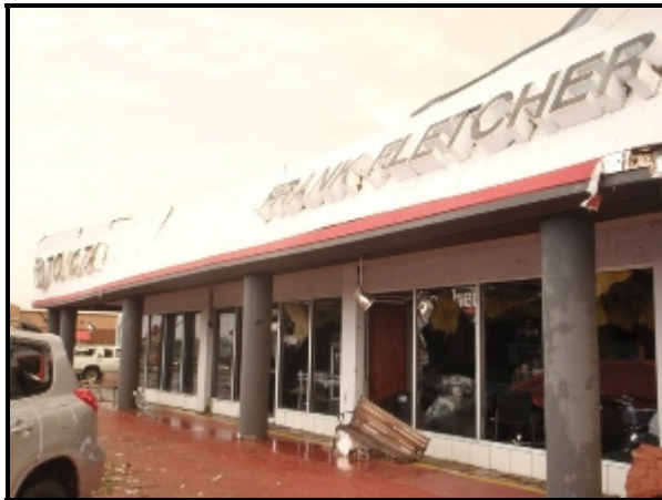
Figure 14. The front (west) elevation of the Fletcher Toyota-Nissan showroom. Flying debris broke the glass windows, and the suspended acoustical tile ceiling fell. This auto showroom was on the south edge of the tornado damage path.
