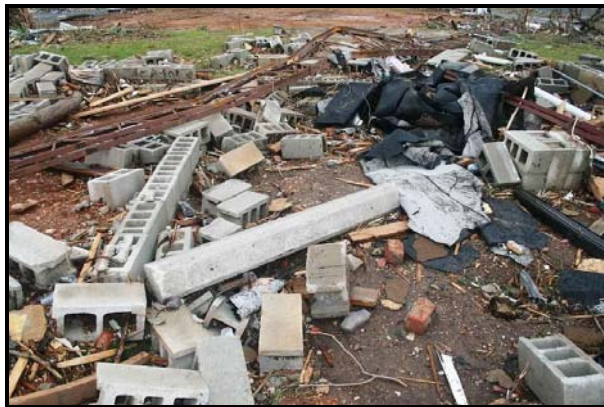
Figure 39. Parking curb found in the crawl space of a destroyed home. The curb traveled 20 m.
