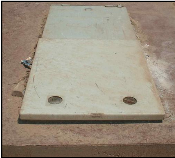
Figure 18. This house had a below ground storm shelter with sliding steel door that was not damaged.
