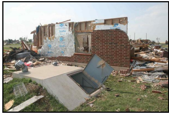
Figure 7. Storm shelter adjacent to a destroyed house. Note the steel door swung outward and had a single, pivoting latch.
