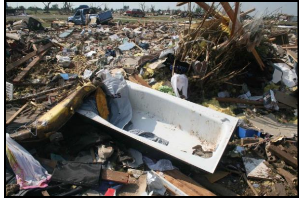
Figure 6. Example of a steel bathtub removed from house foundation. This tub would not have provided adequate shelter during the tornado.
