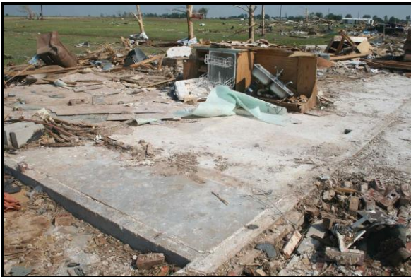
Figure 4. A home nearly swept clean from its concrete slab foundation on Northridge Lane northwest of Piedmont, OK.
