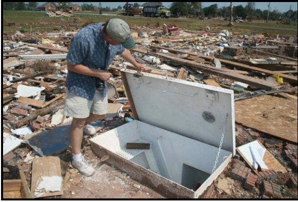
Figure 14. A below-grade steel shelter. The steel door was not damaged.
