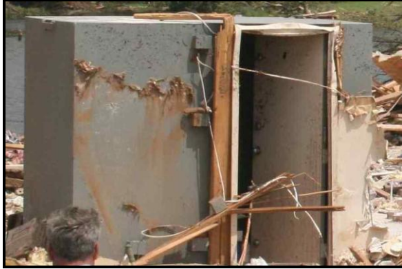
Figure 11. An above ground steel shelter with a steel door survived the tornado.
