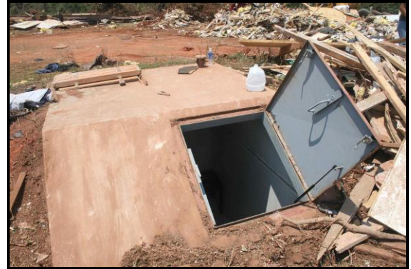
Figure 20. This house had an exterior, below grade storm shelter with steel door that was not damaged.
