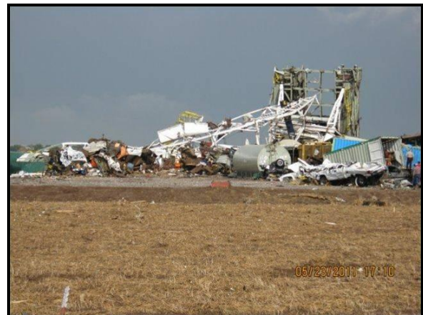
Figure 2. Overturned oil rig at the Cactus 117 drilling site.
