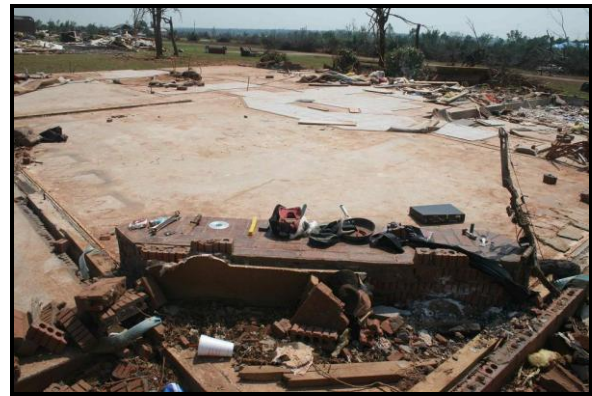
Figure 12. This house was swept clean from its concrete foundation at the intersection of Kitty Hawk Road and Meadowlark Lane.
