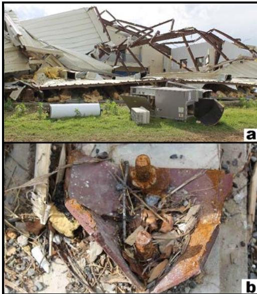
Figure 25. Collapse of this metal church building: a) south wall was pushed inward, and b) torn welds at the base plate. Damage to this building was rated as EF3. However, the adjacent one-story, wood-framed building sustained only EF1 damage.
