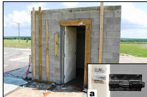
Figure 32. Shelter where six occupants survived the tornado. The substandard door had sliding barrel bolt locks (inset). Fortunately, this door was not struck by wind-borne debris.
