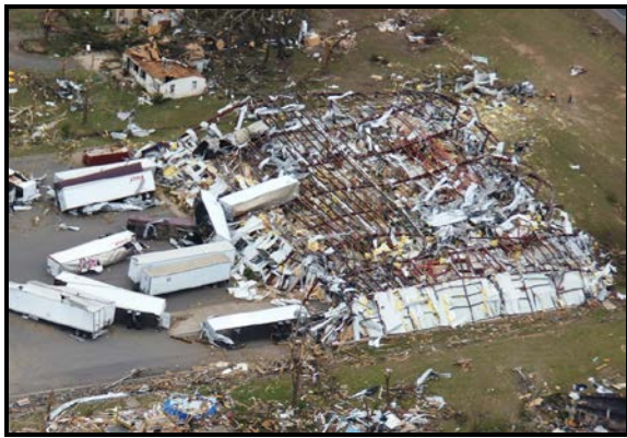
Figure 14. Complete collapse of a metal building with moved truck trailers. Damage to this building was rated EF3.
