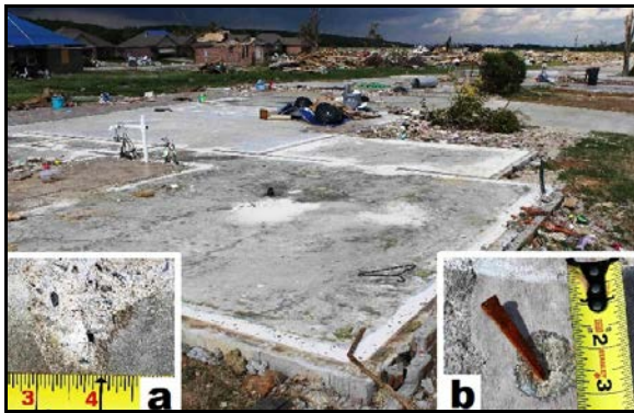
Figure 29. Two modes of failure where cut nails were used to secure the wall bottom plates: a) a nail pulled out of the slab, and b) a wall plate pulled away from the nail leaving the nail bent in the slab.
