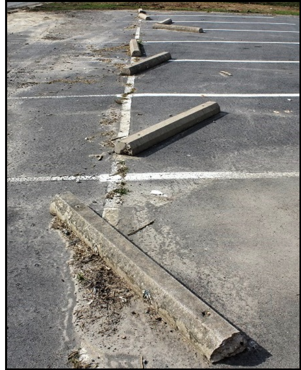
Figure 26. Lateral movement of several unanchored concrete parking stops in front of the Vilonia United Methodist Church. Damage to the main church building was rated EF0.
