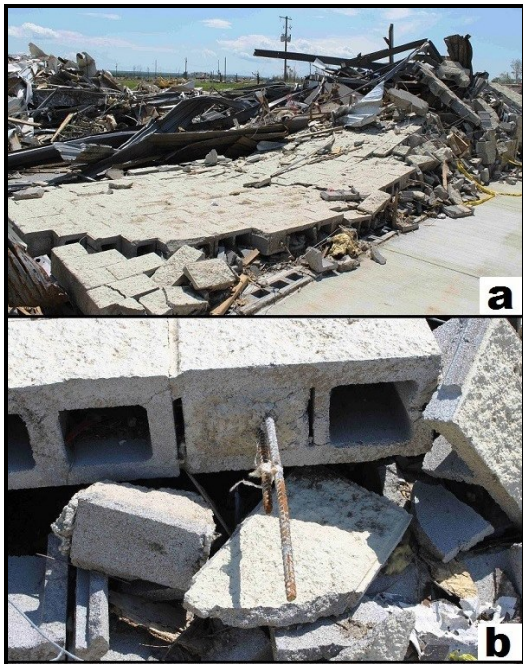
Figure 22. Collapse of a large, isolated retail building: a) wall failure at the top of the slab, and b) foundation rebar pulled out of the CMU foundation. Damage to the building was rated as EF3.
