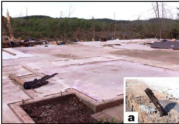
Figure 3. This house was swept clean from its concrete slab foundation as: a) anchor bolts did not have nuts or washers. Because of this deficiency, the unanchored home was rated EF3 instead of EF5.
