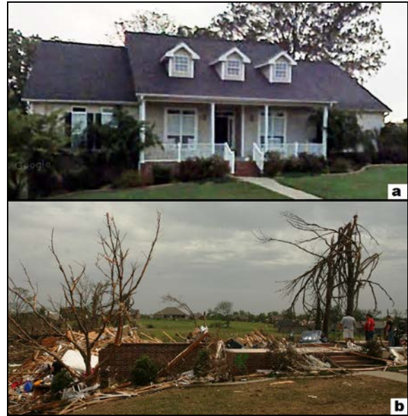
Figure 9. A two-story home: a) before and b) after the tornado. The home collapsed when basement walls supporting the first floor toppled. This home was rated as EF3 damage. The top image is from Google Street View.
