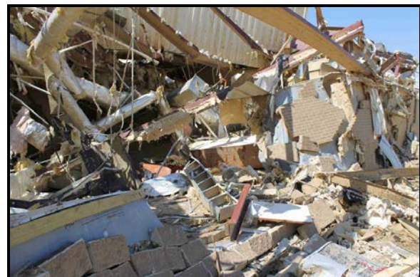
Figure 20. Masonry walls fell into the classrooms on the windward side of the Vilonia Intermediate School. Obviously, these classrooms would not have been places of safe refuge during the tornado.
