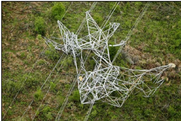
Figure 4. One of several collapsed steel transmission towers that was rated EF-2.
