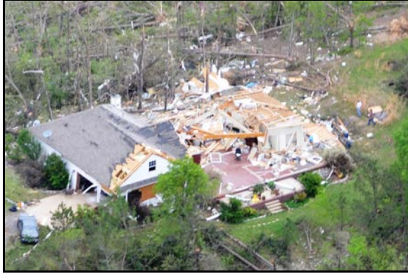
Figure 2. One of the first houses damaged by the tornado lost a portion of its roof and perimeter walls. This home was rated EF2.
