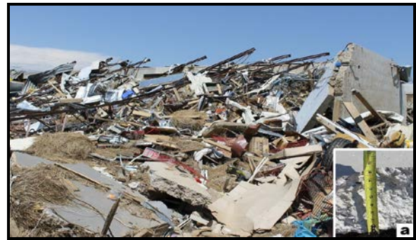
Figure 23. Collapse of the Vilonia Shopping Center constructed with 20 cm thick, poured-in-place, concrete walls. Damage to this building was rated as EF3.
