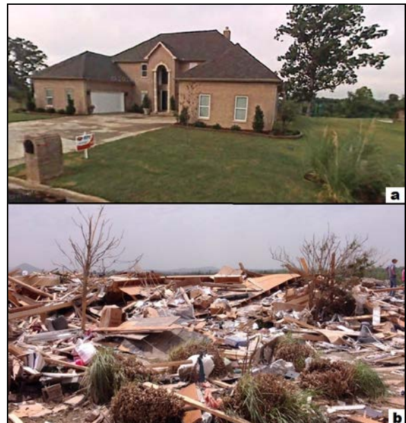
Figure 10. A two-story home: a) before and b) after the tornado. All walls collapsed leaving a pile of debris in the front yard. Damage to this home was rated EF4. The top image is from Google Street View.
