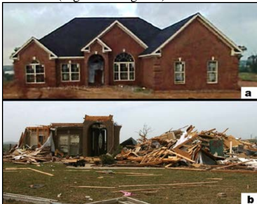
Figure 8. A one-story home: a) before and b) after the tornado. The home was rated EF3 damage. The top image is from Google Street View.
