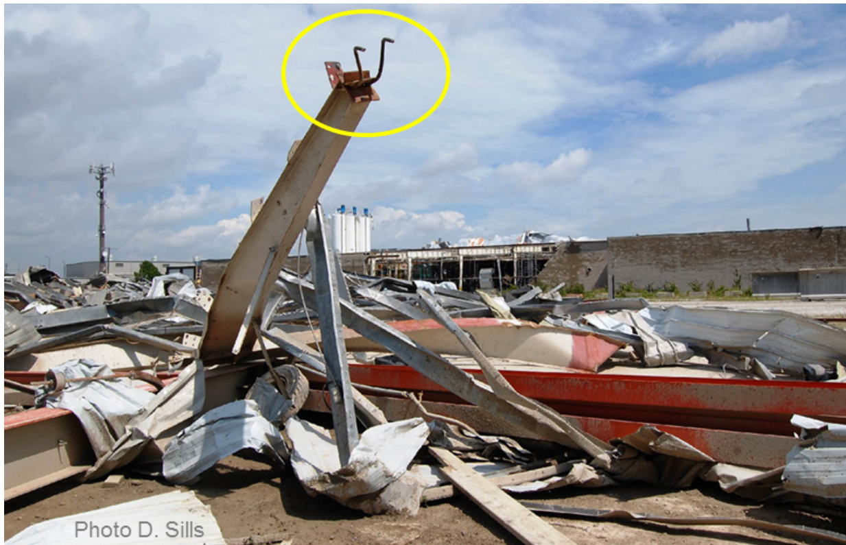
Figure 4. Photograph facing roughly northeast showing EF2 damage, including a metal warehouse that collapsed completely and was partially moved off its foundation. Premature material failures were found to have occurred at the connections between the foundation and the bases of the columns (one of which is circled in the photograph).
