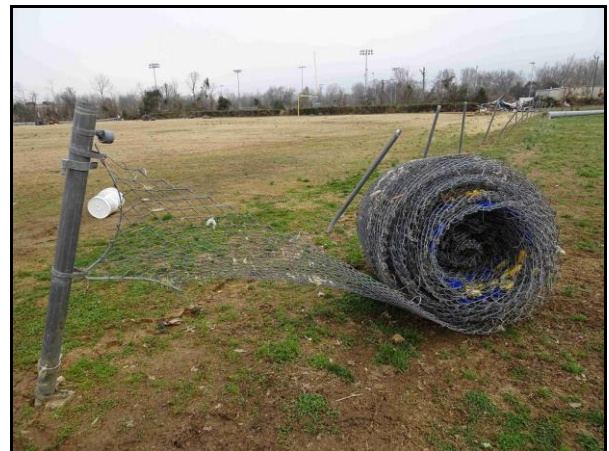
Fig 20. Rolled up chain-link fence at West Wilson Middle School.
