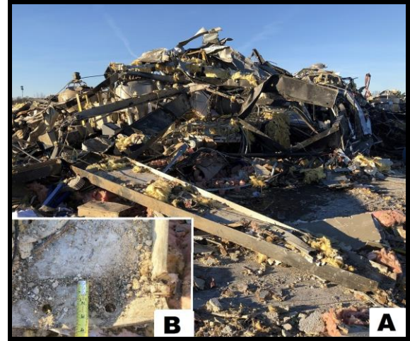
Fig. 14. Collapse of the Candle Factory building: A) pile of steel debris on the foundation with support column in foreground, and B) closer view showing bent base plate on column where it had been bolted.
