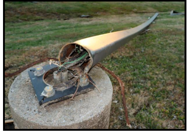
Fig. 18. A steel light pole tore at its base near Pilgrim Pride north building.
