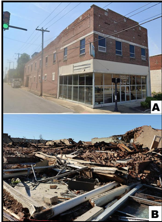
Fig. 11. Midstate's Glass Company building: A) Google Street View before the tornado, and B) complete collapse of building from the tornado.
