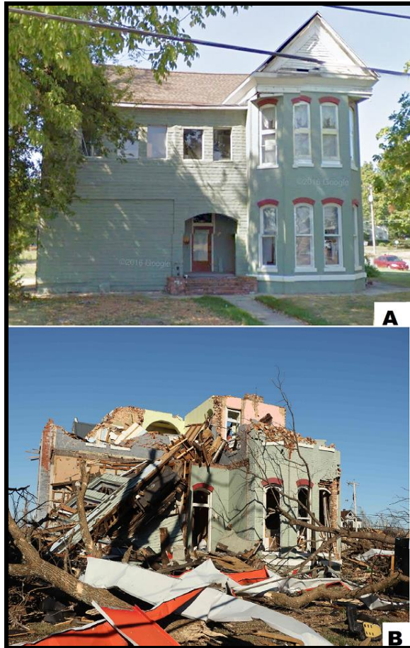
Fig. 6. Two-story wood-framed residence clad with brick masonry: A) Google Street View before the tornado and B) view of house after the tornado.
