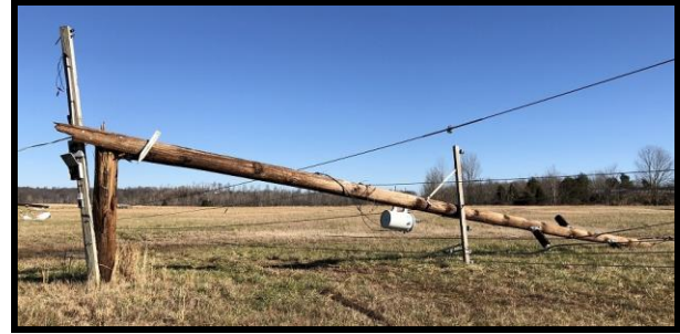
Fig. 16. Broken wood power pole.
