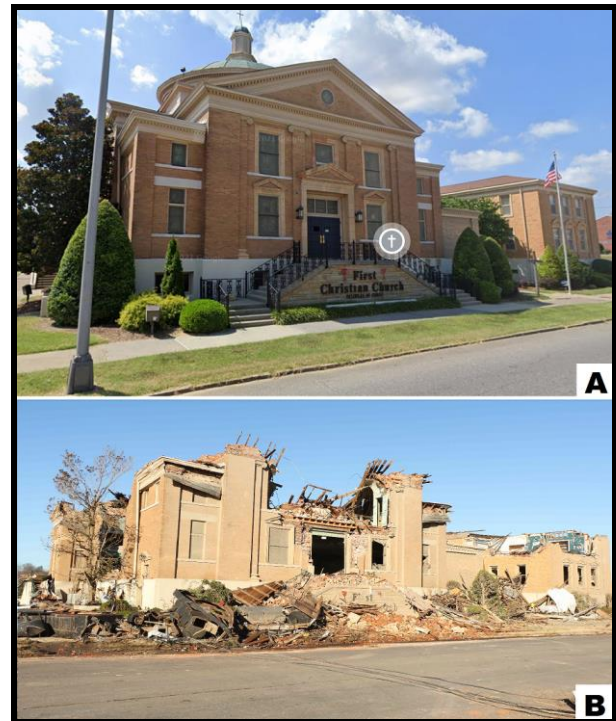
Fig. 20. First Christian Church in Mayfield: A) Google Street View before the tornado, and B) collapsed domed roof and top story after the tornado.
