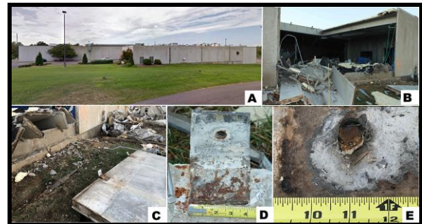
Fig. 12. Pilgrims Pride building: A) Google Street View before the tornado, B) loss of two wall panels from the tornado, C) closer view of the base of the toppled wall panel, D) steel bracket embed remained intact on the wall panel, E) broken anchor bolt in the foundation.
