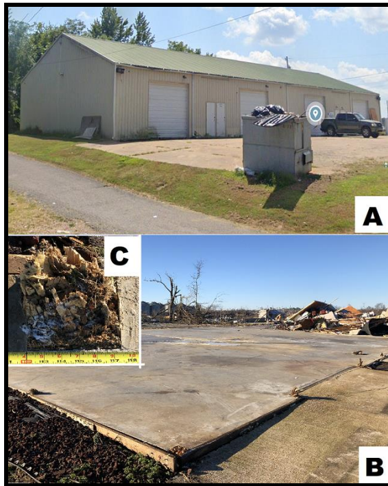
Fig. 4. Wood post and frame building in Mayfield, Kentucky: A) Google Street View of front (north) elevation before the tornado, B) building view after the tornado, and C) wood post snapped at foundation.
