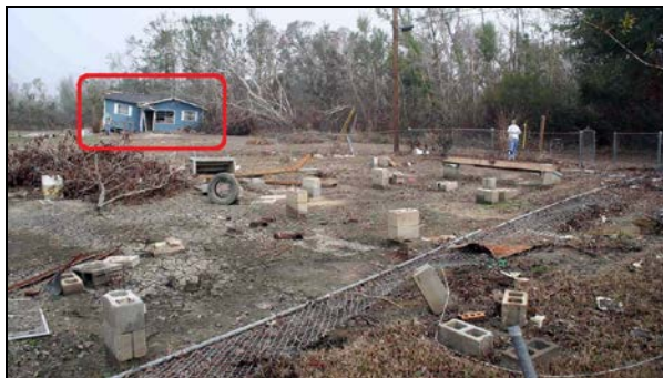
Figure 3. This wood-framed house (red outline) floated landward from its stacked CMU foundation (foreground) where it was stopped by trees in Pass Christian, MS. The home was not picked up and transported by a tornado as some have argued.
