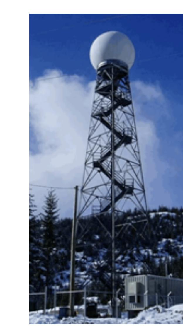
UHF-band radar wind profiler
