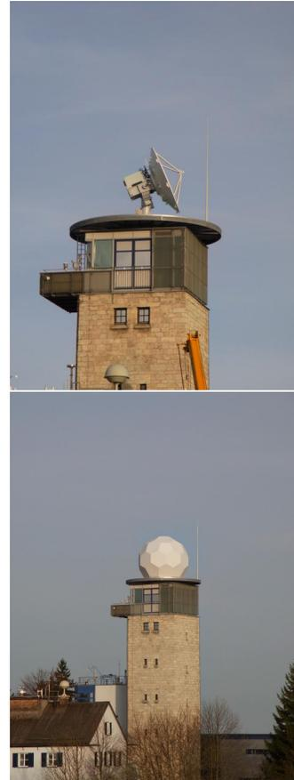
Figure 1: Radar system during a pattern test in April 2011, upper picture without the radome, lower picture with the new radome.
