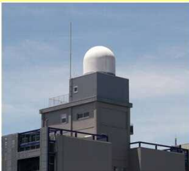
Phased-Array Antenna System of X-band PAWR
