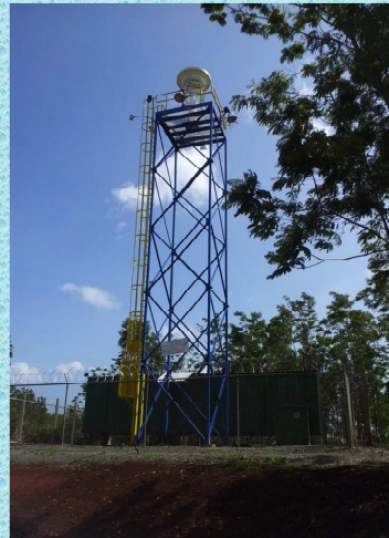
Tropinet-1: An X-band Dual-Pol Doppler Radar node at Cabo Rojo, PR
