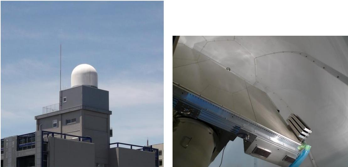
Fig. 1 Phased Array Radar at the top of the building in Osaka University.
