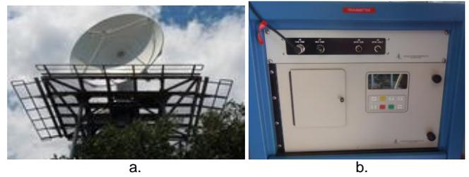
Fig. 3. a. Parabolic reflector and b. magnetron transmitter of Torchiarolo radar.
