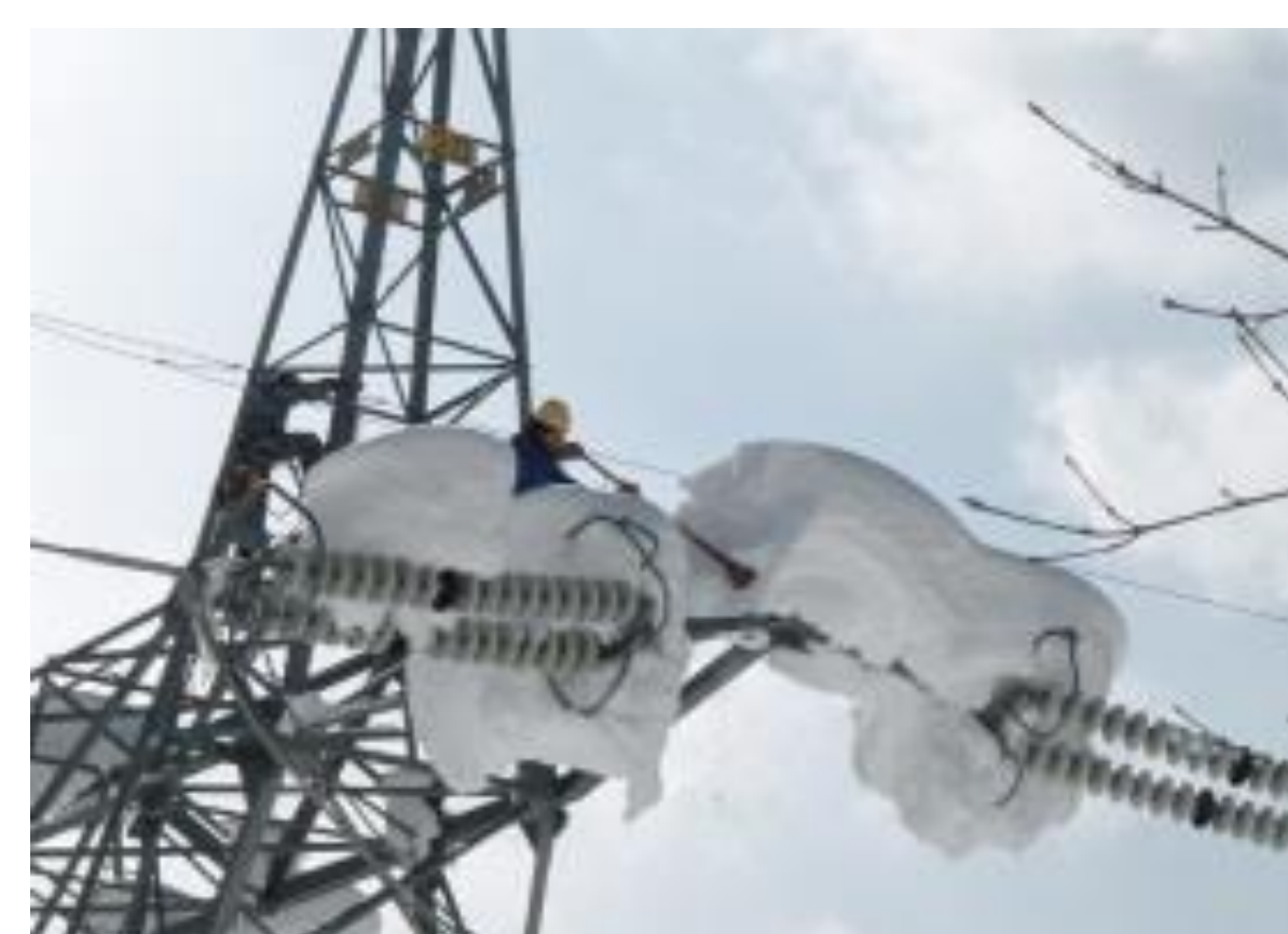
Fig.1 Snow on the electric power line.
