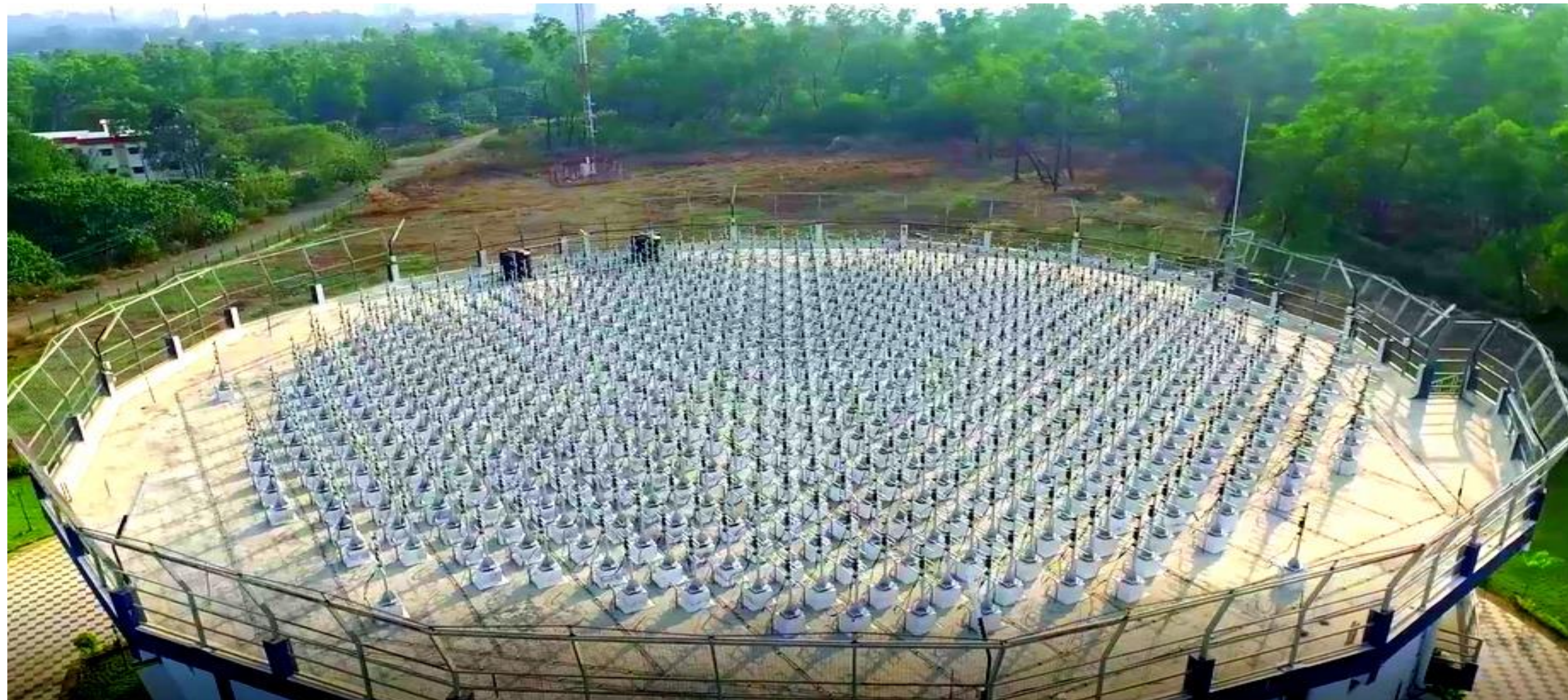
Fig. 1: An aerial view of the 619 element 205 MHz Wind profiler Radar atop the ACARR institute at Cochin.
