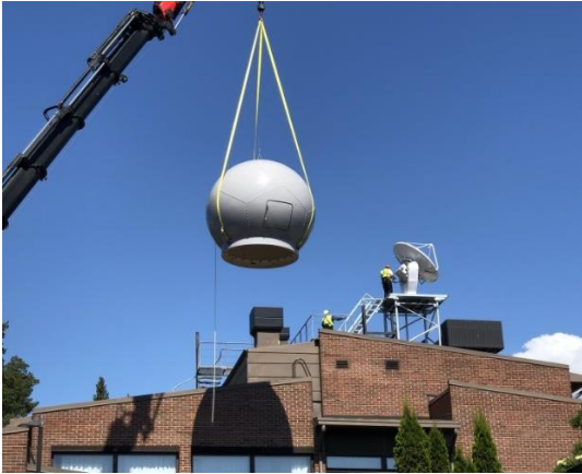
Figure 4. Research WRS400 used in this study was installed in summer 2020. It is located at the roof top of Vaisala headquarters, 12km north of Helsinki, Finland. This radar is equipped with 2.4m antenna (Picture P. Puhakka).
