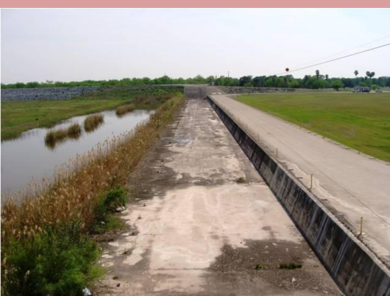
Banker floodway before diversion at Anzalduas
