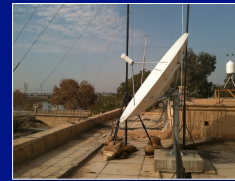
EUMETSAT reception dish installed and operational
