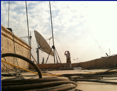
An IPSM technician makes final adjustments to the EUMETSAT reception dish
