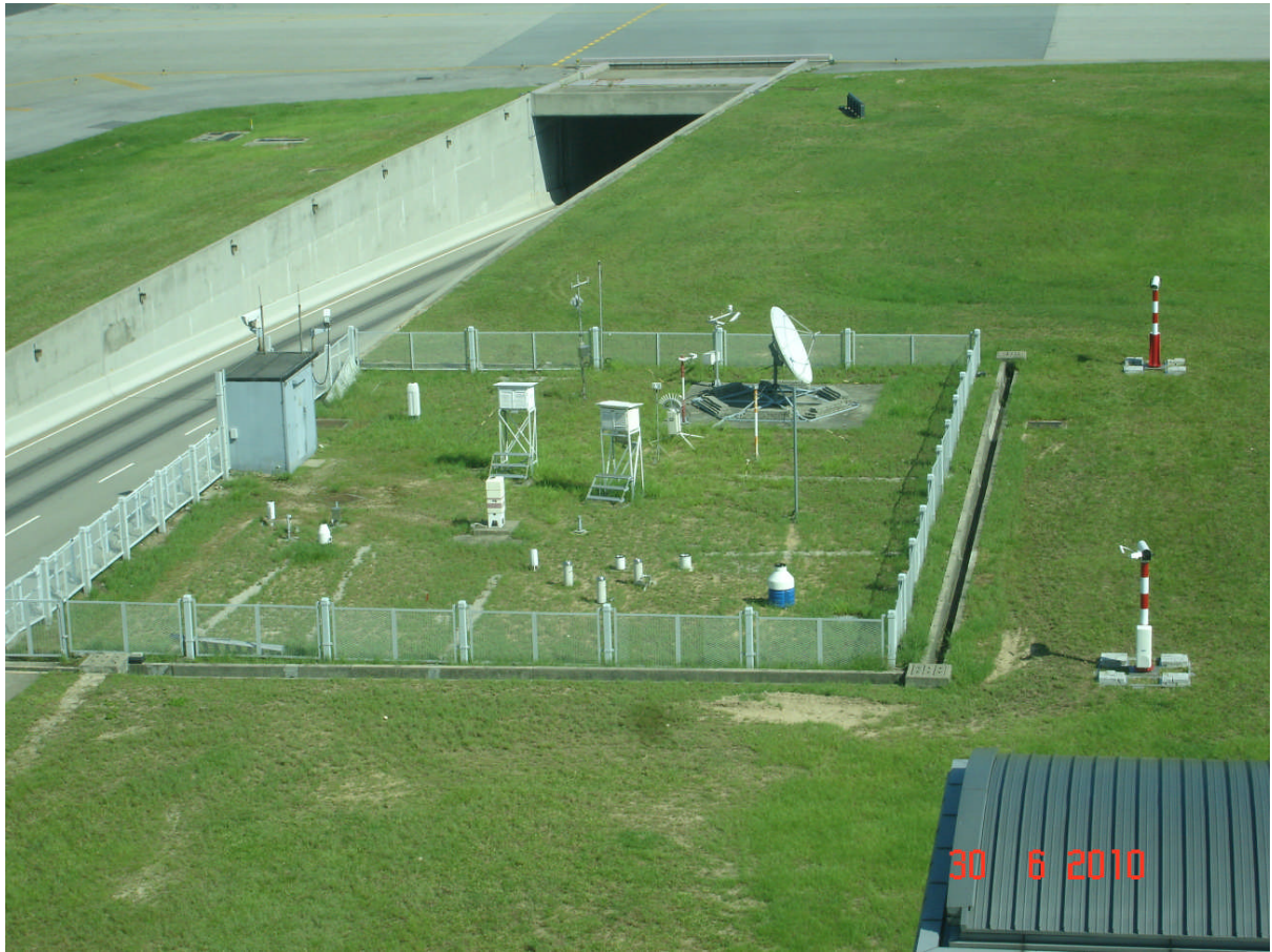
Figure 1 Setup of the rain gauges at the Hong Kong International Airport
