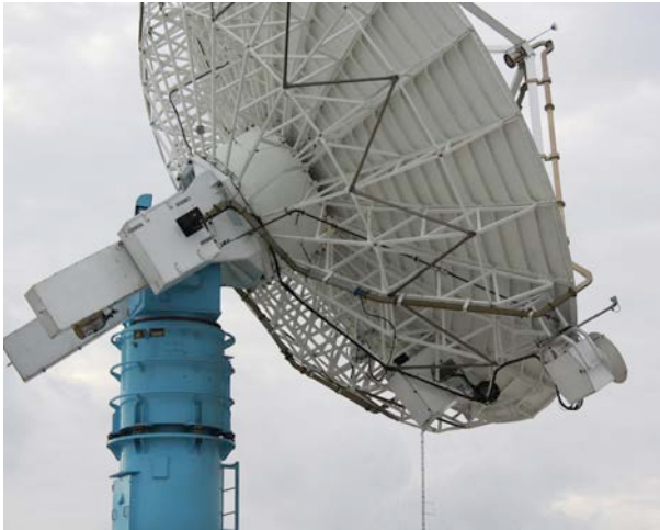
Figure 6. The large S-Band antenna carrying the smaller Ka-band antenna on the lower right.
