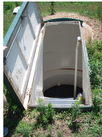
Fig. 3. In ground shelter where a family in Rainsville survived as an EF-5 destroyed their home (also note scouring to grass that had covered the top portion of the shelter). Visual observation of the tornado prompted sheltering action, as the widespread power outage made obtaining updated weather information difficult.
