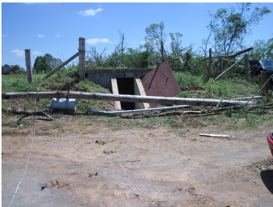
Fig. 2. A downed telephone pole blocked the only entrance/exit of a storm shelter where a dozen friends and neighbors survived in Lawrence County. They were trapped until two men inside were able to shove the door open enough to knock the pole forward.
