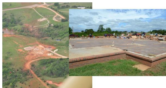
Figure 8: Aerial and ground photographs of a home which was removed from its foundation towards the end of the Goldsby tornado path.
