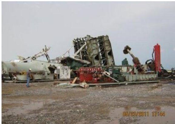
Figure 9: Cactus Rig 117. The base of the rig can be seen in the middle of the image, with the mast lying towards the left and behind the tank on the left. The blowout preventer is seen in the foreground just to the right of the rig. Photo courtesy Derrick Brown
