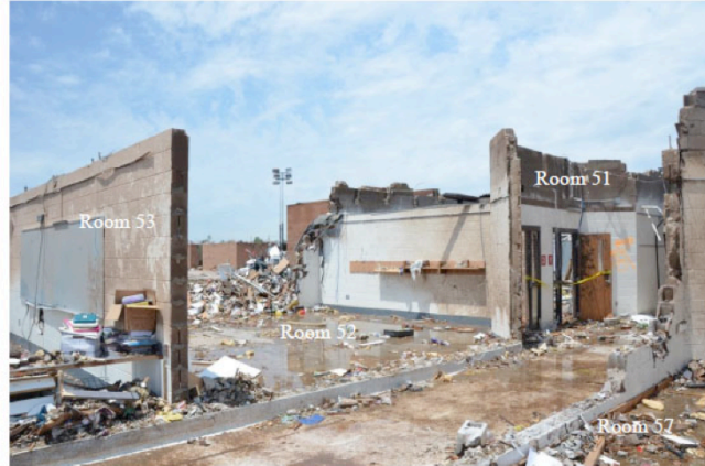
Figure 4-6. Damage to the hallway and classrooms of the new main classroom building (complete loss of roof and many walls) where the 7 fatalities occurred (most of the debris has already been removed). This hallway area was a “designated area of safety.”
