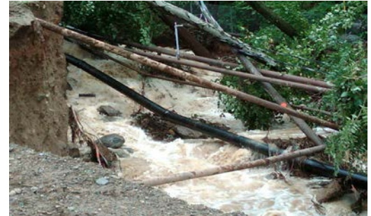
Transmission main washout Photo courtesy of Jim Glozzy
