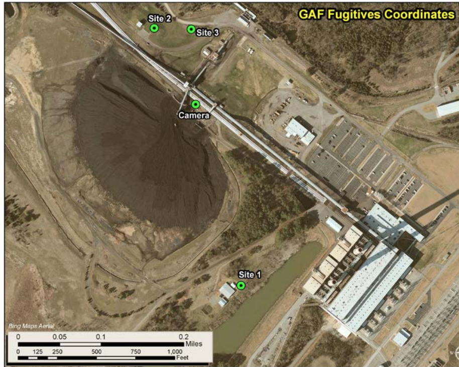
Figure 1. Environs surrounding the coal pile (oval black area) at the Tennessee study site. The photograph is oriented north-south from top to bottom. Monitoring sites are denoted by green circles.
