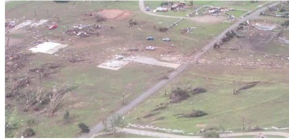
Figure 6: Aerial image of swept foundation. Ground surveys found that the home was only secured to the foundation using cut nails, resulting in EF4 rating.
