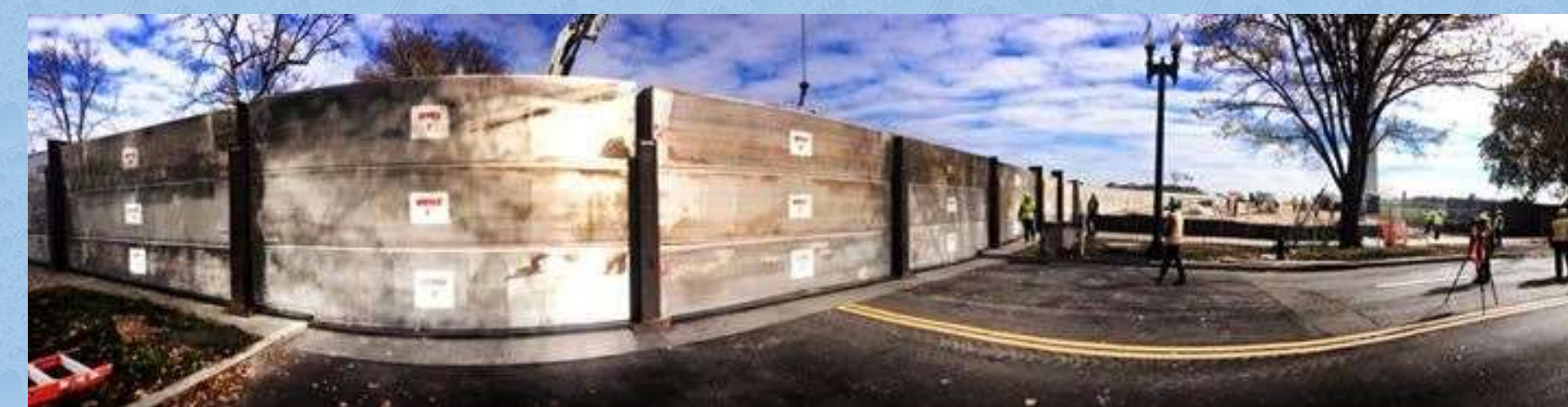
Test Installation of 17 th Street Closure, Washington, DC, on October 31 st 2014. Photo courtesy U.S. Army Corps of Engineers.
