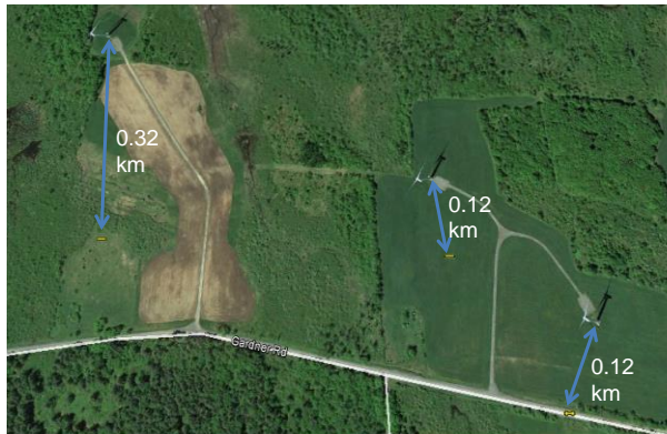
Figure 12. Google Earth image showing turbines and ENTLN-detected flashes. The Ruler tool was used to calculate the distance of the nearest flash to the turbine base.
