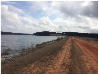
Earthen dams backing up tribal reservoirs (Pushmataha Dam, MS pictured) are at risk due to heavy rain events. A heavily traveled road lies just downstream of this dam, so dam failure would impede traffic in the region and potentially place drivers at risk (Nixon 2015). Timely forecasts of heavy rain events would help reduce this risk.
