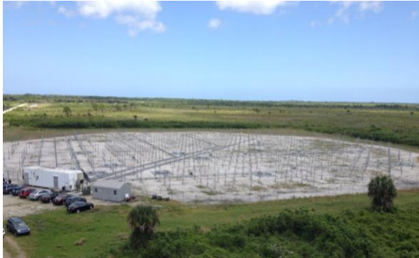
Figure 1. Aerial view of NASA KSC TDRWP. System electronics are housed in trailer on the bottom left of photo.
