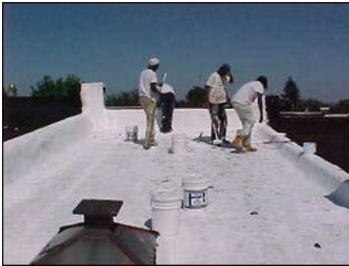
Figure 2. Workers apply a cool roof coating on a rowhouse in Baltimore, MD (courtesy EPA HIRI web site).
