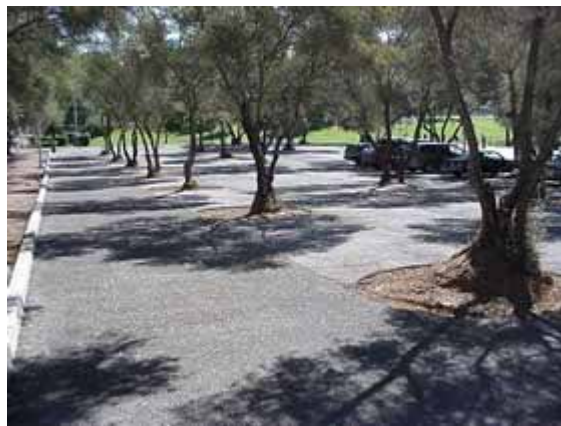
Figure 3. A pervious lot in Fair Oaks, California's Miller Park with 23 mature Olive trees, which provide shade and give the parking lot a natural look (courtesy, US EPA, HIRI web site).
