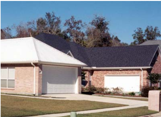
Figure 4. Example of a lone high albedo roof in an otherwise dark-roofed residential neighborhood in New Orleans (photo by D.J. Sailor).
