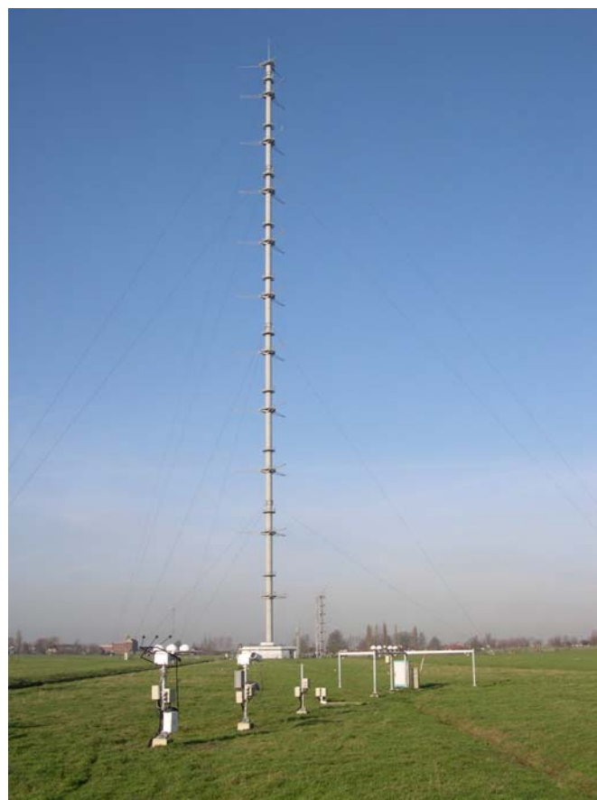
Figure1. The 213 m meteorological tower at Cabauw, The Netherlands.
