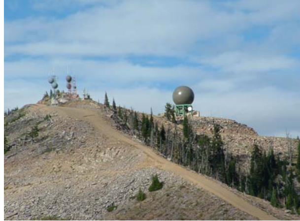
Figure 1- The Missoula, Montana WSR-88D radome is about 4600 feet higher than nearby populated valleys and nearly 8000 feet above sea level.
