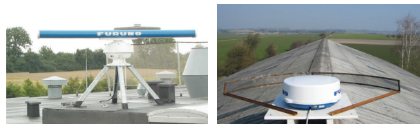
Figure 2 Example of LAWR installations. The LAWR on the left is a standard LAWR. The one on the right is a City-LAWR. Besides the antenna unit on the image there is a small cabinet with two PC's and the radar control unit.
