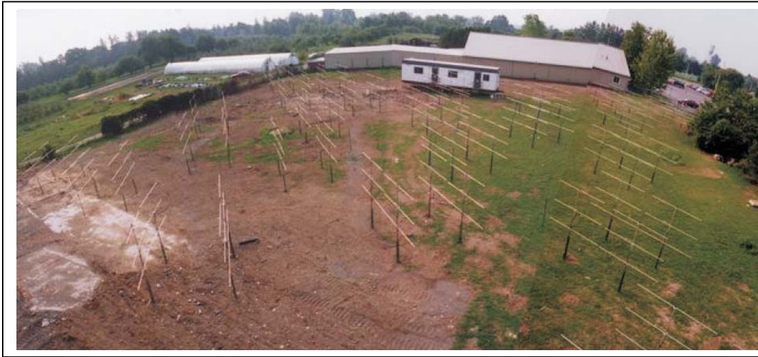
Fig. 3. Aerial view of the McGill radar during construction
