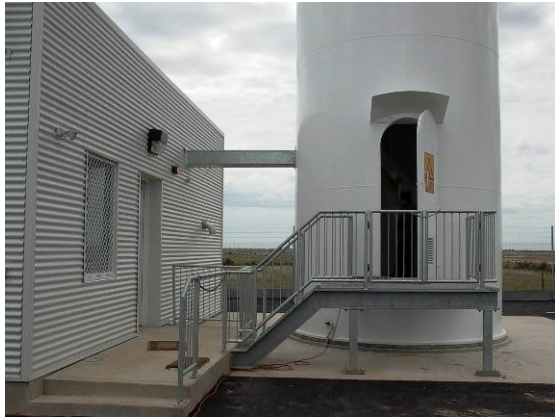
Figure 2 – Tower Base/Entrance and Radar Shelter
